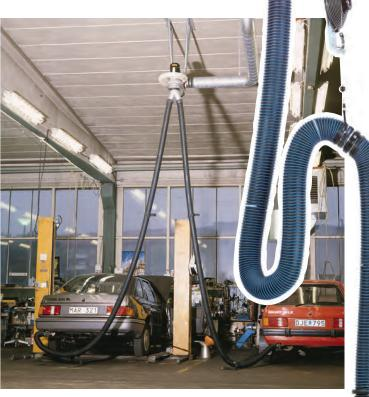
The single exhaust extractor is a reliable and functional solution for all types of stationary vehicles. Available with balancer or a cord for manual hose suspension. The balancer automatically raises the hose and nozzle after disconnection, and keeps them lifted clear of the floor at all times. Models for high temperature application are available.
